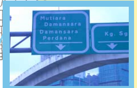
Penchala Link Highway
